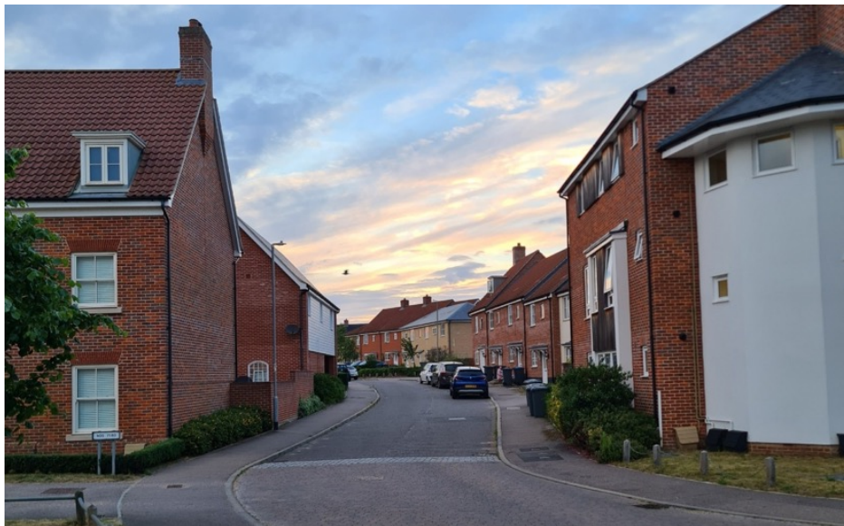
An example of poorly integrated affordable home, with a clear differentiation in style and material palette. (Credit: Create Streets)
