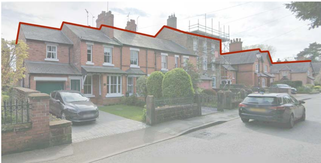
The mix of building types and heights creates a varied roofline with an organic feel, Pepper Street, Christleton
