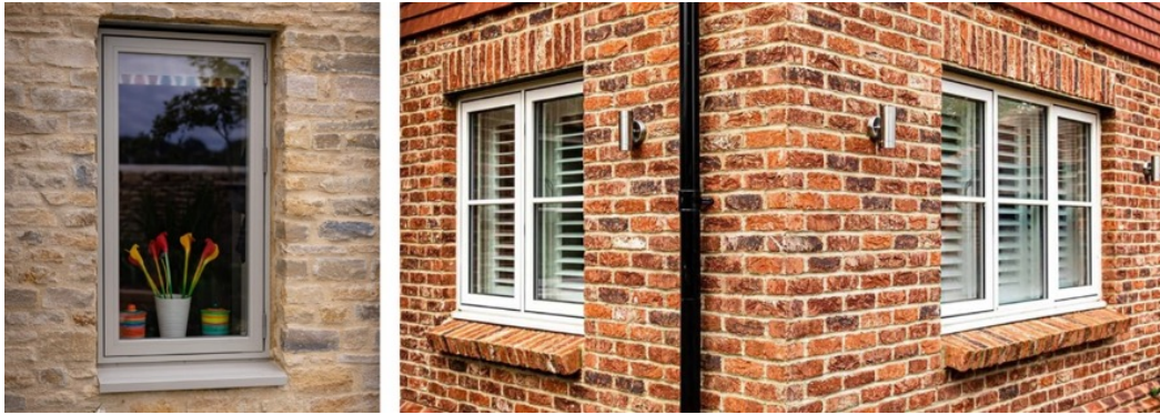
Examples of triple-glazed casement windows which meet Passivhaus U-values
