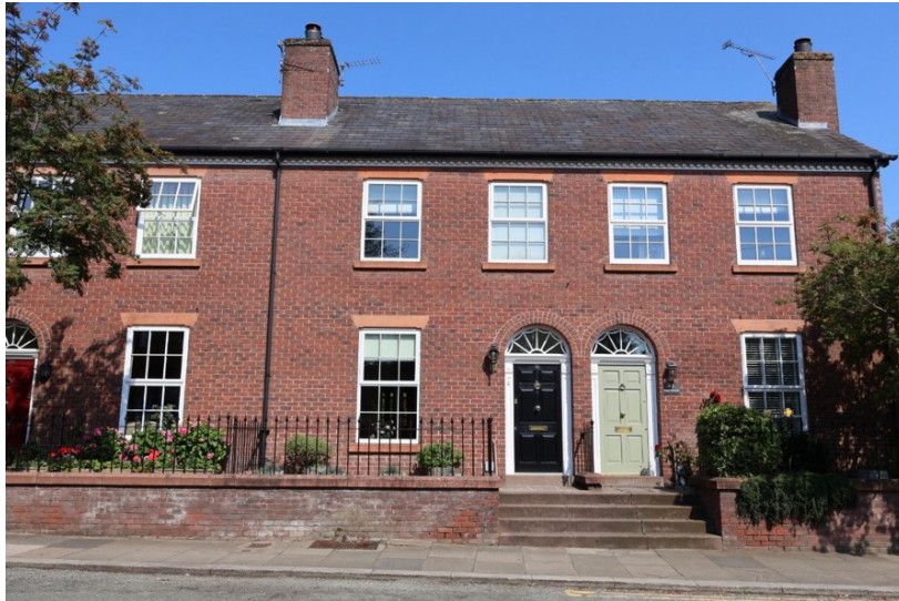
Example of newly built, simple, Cheshire vernacular terraces, Tarporley. (Credit: Create Streets)
