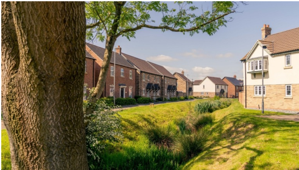
A swale within a green corridor in a development in Alford, East Lindsey, Lincolnshire (Credit: Lincolnshire County Council)
